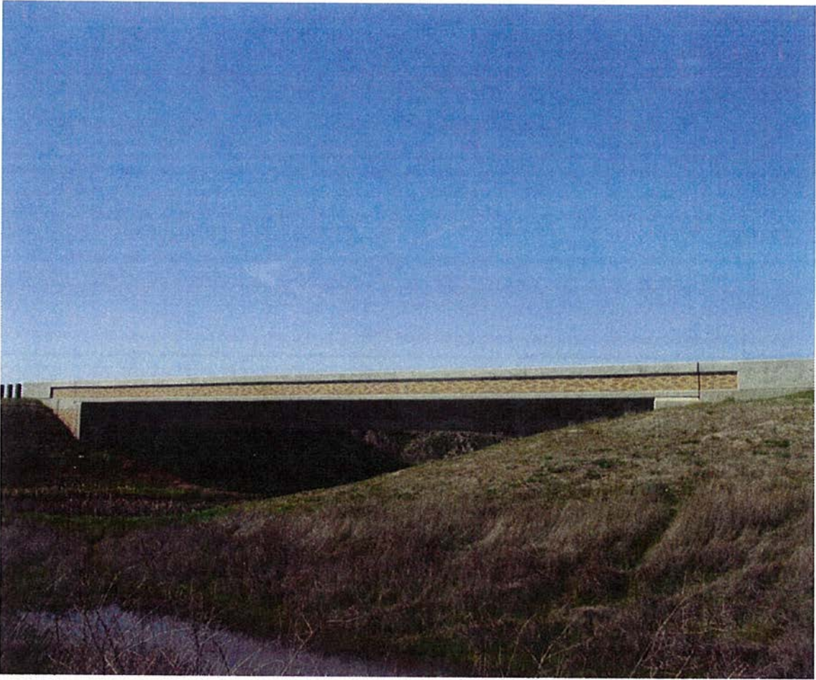
NORTH YANKEE SLOUGH BRIDGE RIGHT - LOOKING WEST
